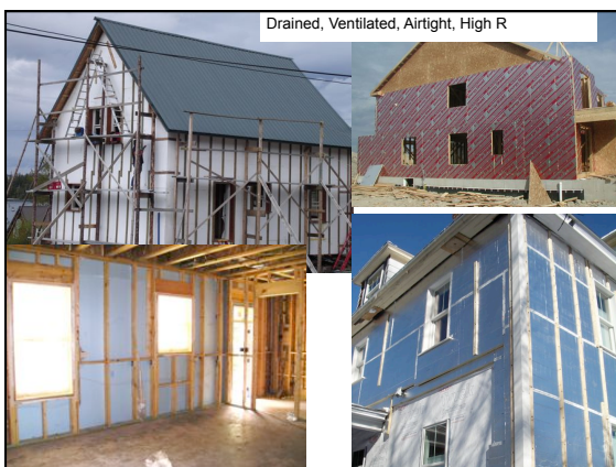
Drained, Ventilated, Airtight, High R
