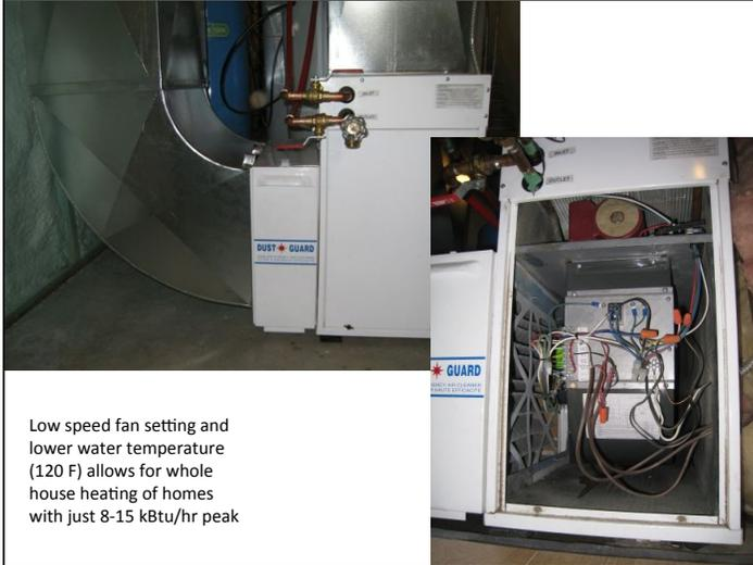
Low speed fan setting and lower water temperature (120 F) allows for whole house heating of homes with just 8-15 kBtu/hr peak
