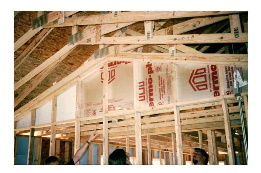
Tall 2x6 walls bow outwards during the winter...due to the temperature difference leading to a relative humidity difference...
