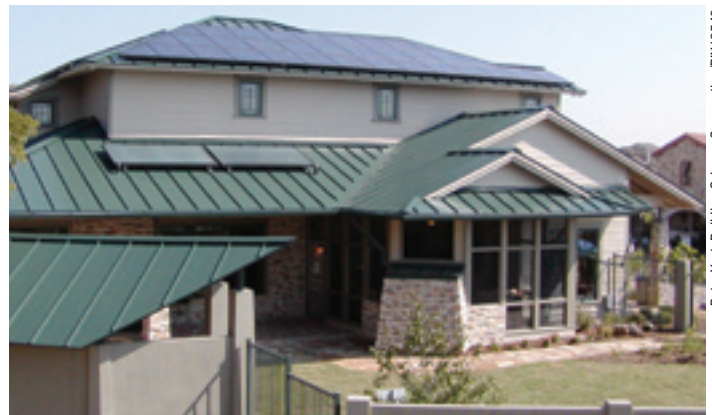
Great unobstructed southern exposure for the photovoltaic and solar water panels, the “engines” of this Zero Energy Home.
