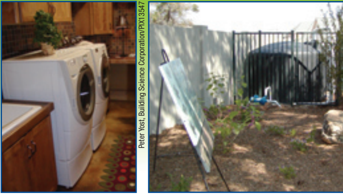
From the inside—H-axis clothes washer—to the outside—rainwater cisterns—this home is a water miser.
